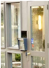
Bldg E entry
