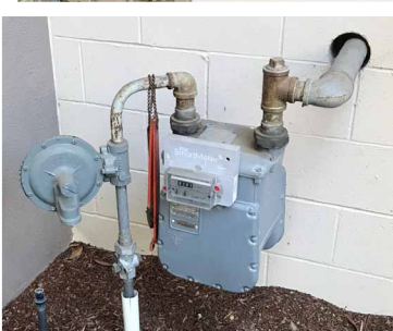
To the right of Bldg E entrance in corner. Wrench at gas meter.
