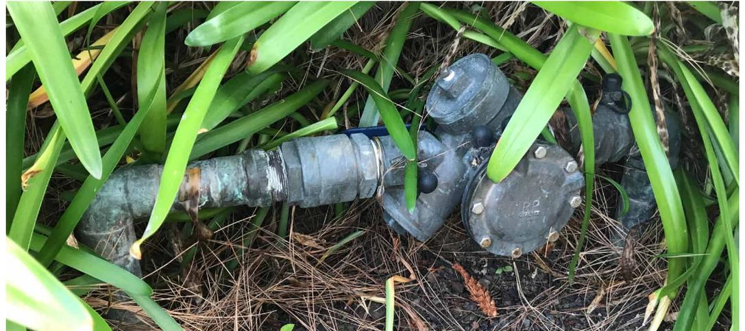
**Valve handles aligned, horizontal: Valves open.
